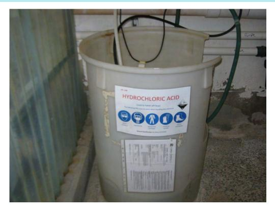
**Photograph 7:** AEC 2 – Large quantity of chemicals stored in the outdoor pool plant room.
